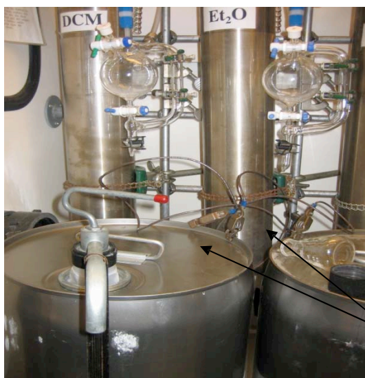
Bonding wires between drums
